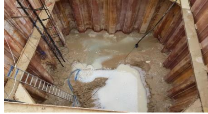
d) Protection for construction pit
